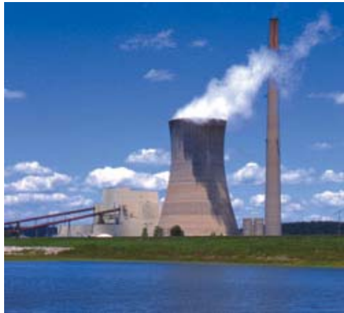
Mountaineer Plant - New Haven, WV
